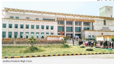
Andhra Pradesh High Court
